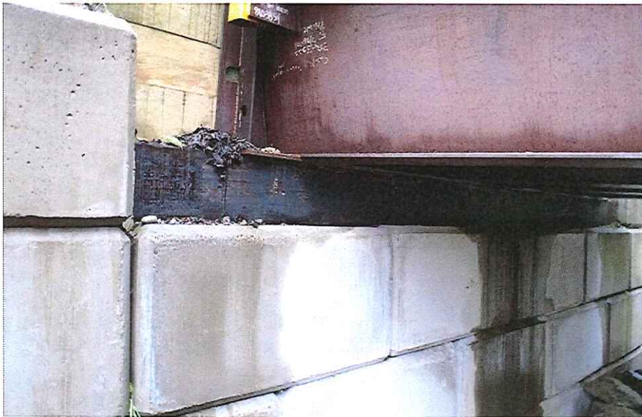
CK2103 Right Abutment SIII
