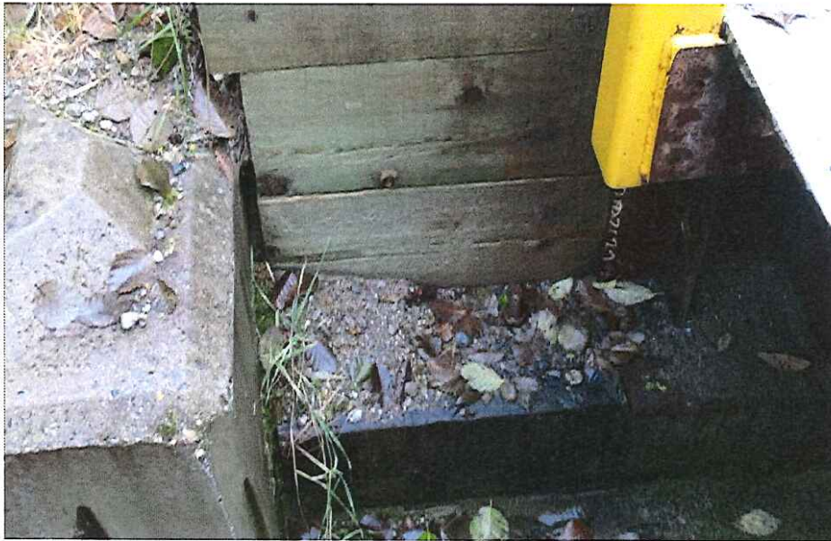
CK2103 Left Abutment Sill
