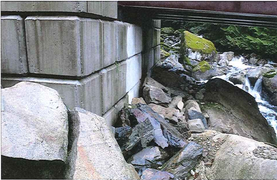
CK2103 Right Abutment
