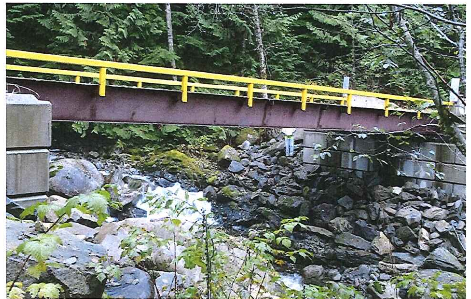
CK2103 From Downstream
