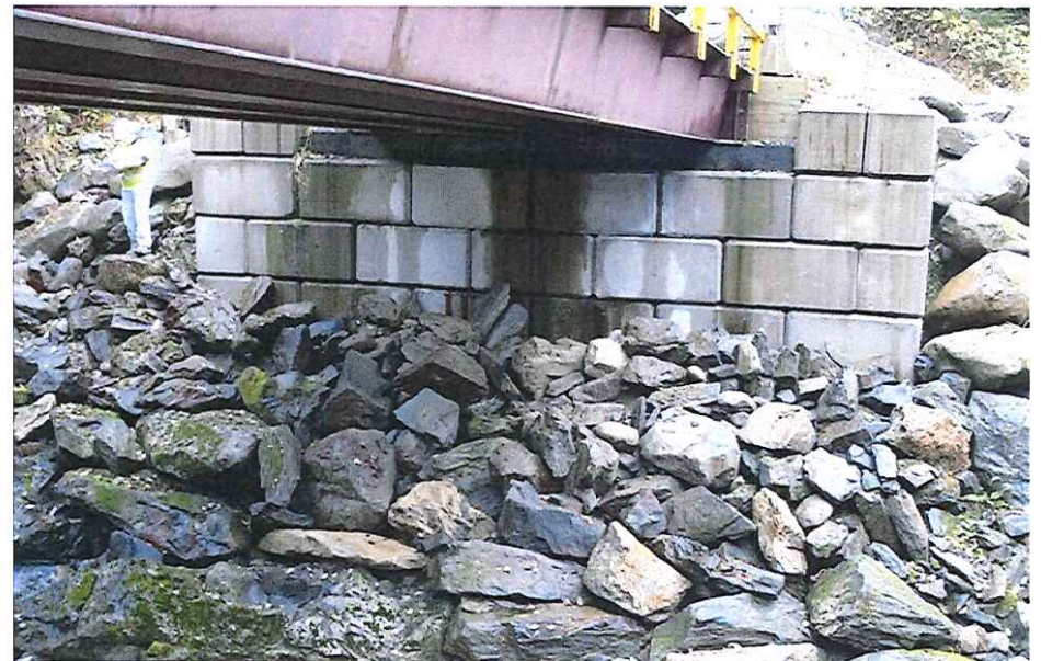
CK2103 Left Abutment
